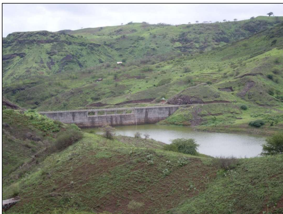
Figure 43 Poilão Dam, a critical component of Santiago's surface water infrastructure. Source 148 .
